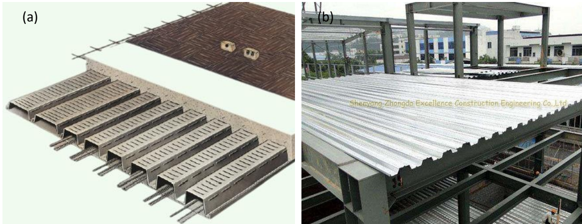
Figure 2.4: Panels corrugated profiles (a) with concrete [1], (b) without concrete ( https://www.prefabricatedsteelstructures.com/sale-9458035-aisi-astm-corrugated-steel-floor-decking-sheet-steel-structure-0-5mm-1-2mm.html [accessed on November 2024]).
