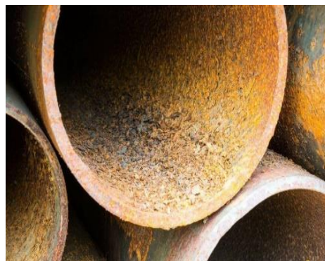
Figure I.8. Corrosion inter granulaire [34].
