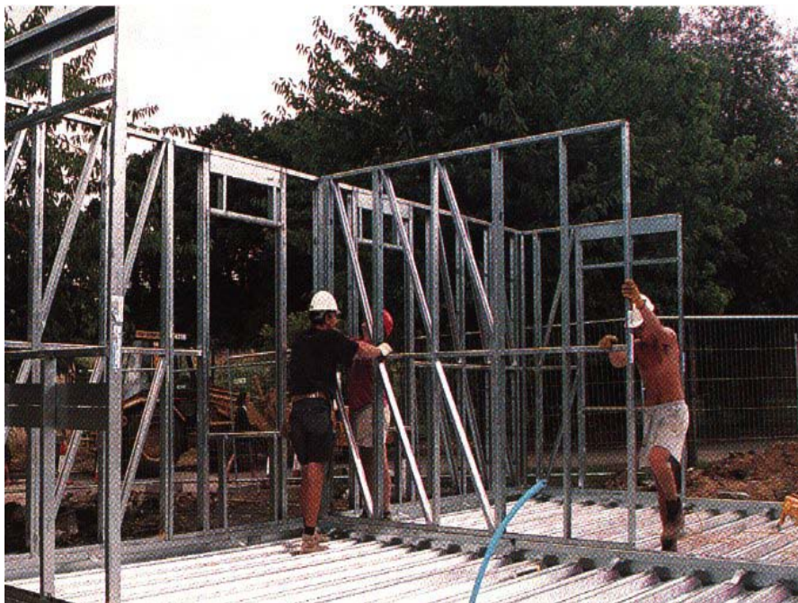
Figure 4.1 typical light steel structure assemblies.
