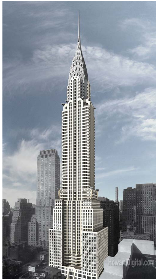
Fig 1.3; Chrysler Building Designed by Willian Van Allen and opened on 27th May 1930.
