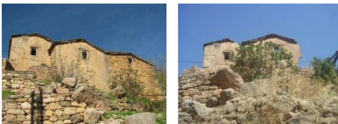
Figure 1: Left, photograph of a traditional building taken in 2012 (source: PPSMVSS diagnostic report). Right, photograph of the same building taken in 2016 (source: study report by Frendi Karima).
