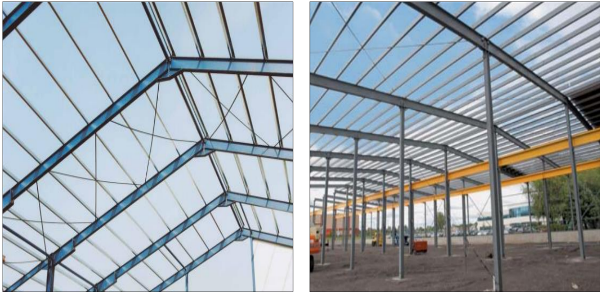
Figure I.4. Cold-formed steel profiles used as purlins and cladding rails.
