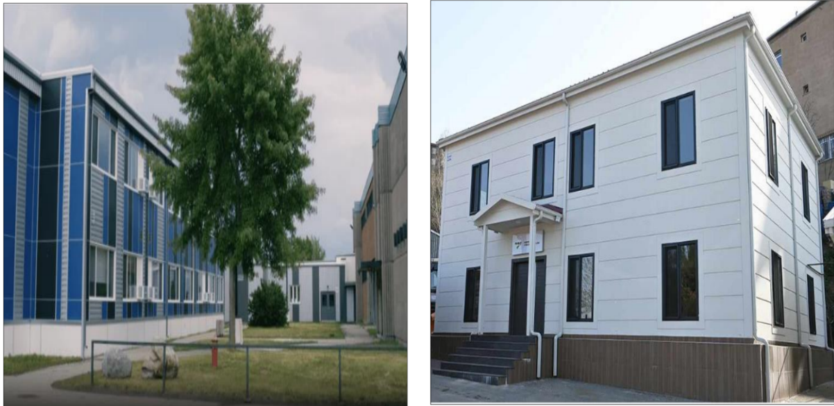
Figure I.12. Prefabricated modular units used for buildings, schools, and offices.
