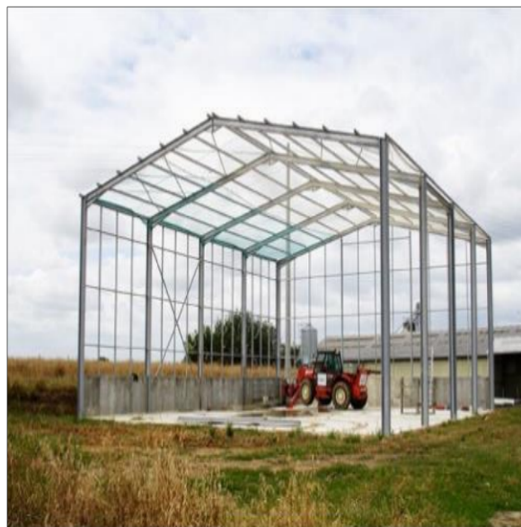
Figure I.5. Cold-formed steel framing.
