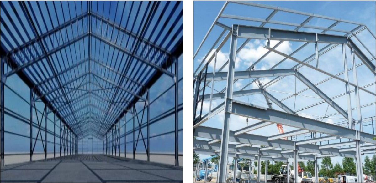
Figure I.10. Roof truss using C-sections.
