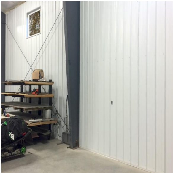
Figure I.8. Wall panels made of cold-formed steel profiles.
