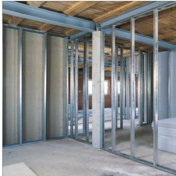
Figure I.6. Cold-formed steel partition walls.
