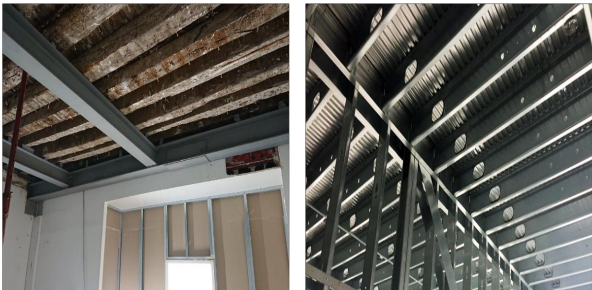
Figure I.7. Floor joists made of cold-formed steel.
