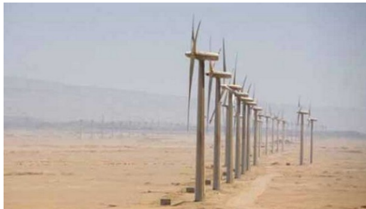
Figure 5.4: Kabertene wind farm (Khadir and Bouziane 2020)
