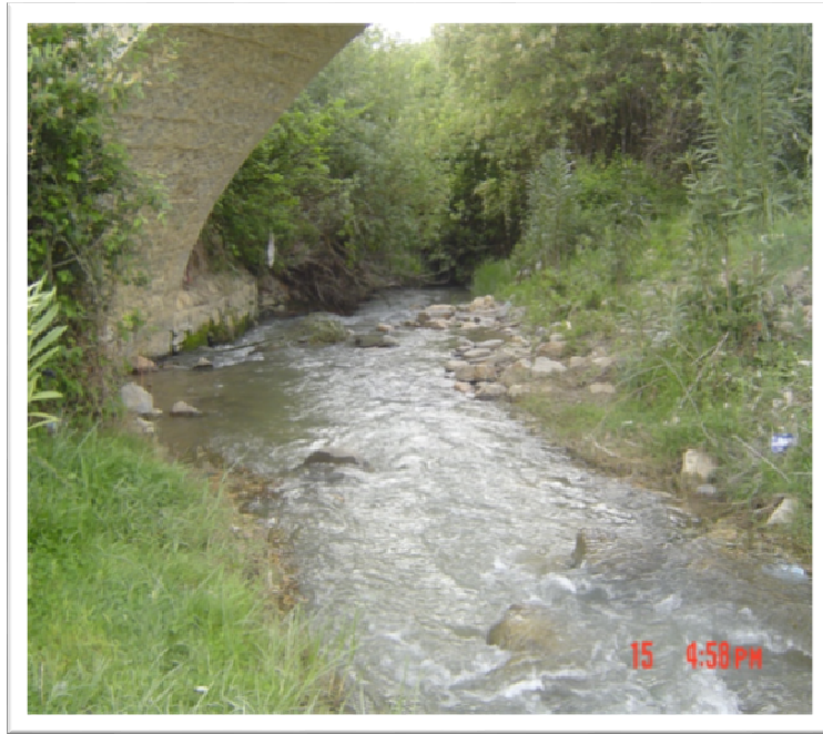
Figure 31. Station Oued Cheniour (cliché Bouhala, 2008).
