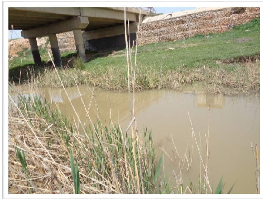
Figure 25. Station Pont Sedrata 1 (cliché Bouhala, 2008).
