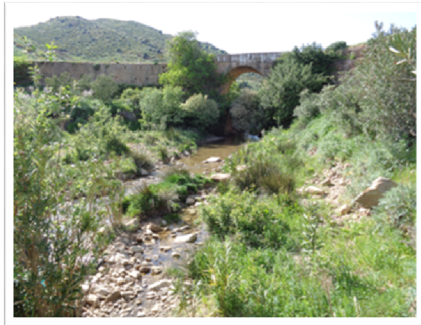
Figure 18. Station de Bou El Frais (cliché Bouhala, 2014).
